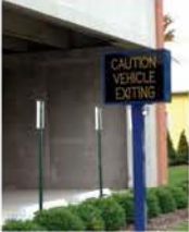
Exiting vehicle signage, sensors, and warning indicators (Located at both west and south vehicle entrances/exits)
