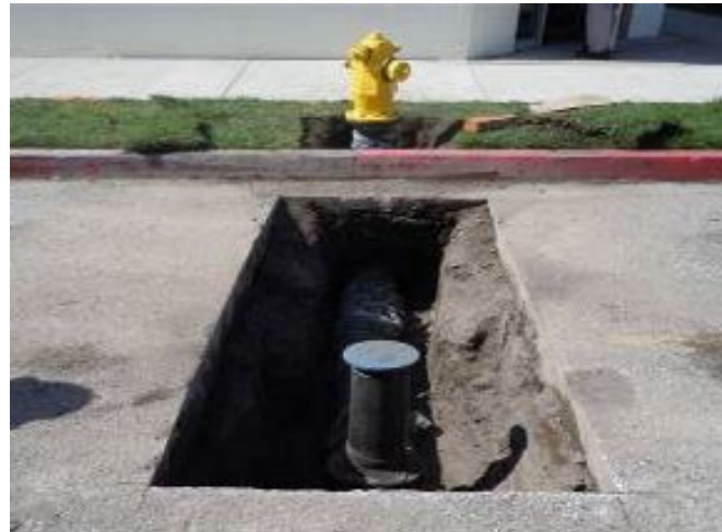
Fire hydrant reconnection
