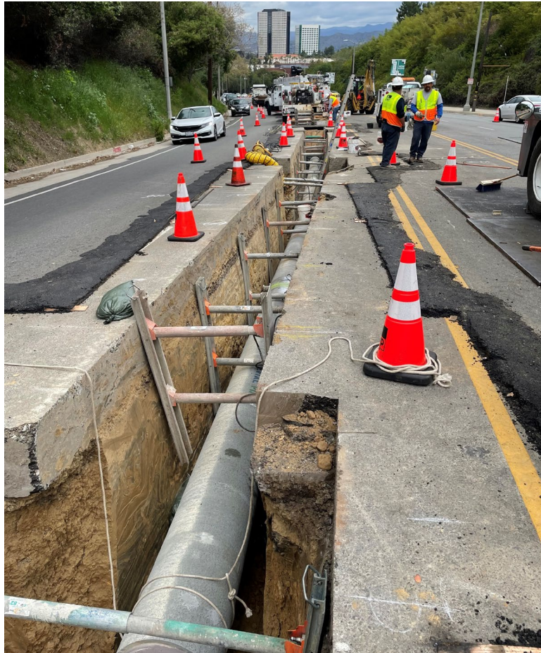
Daily mainline traffic setup/removal
